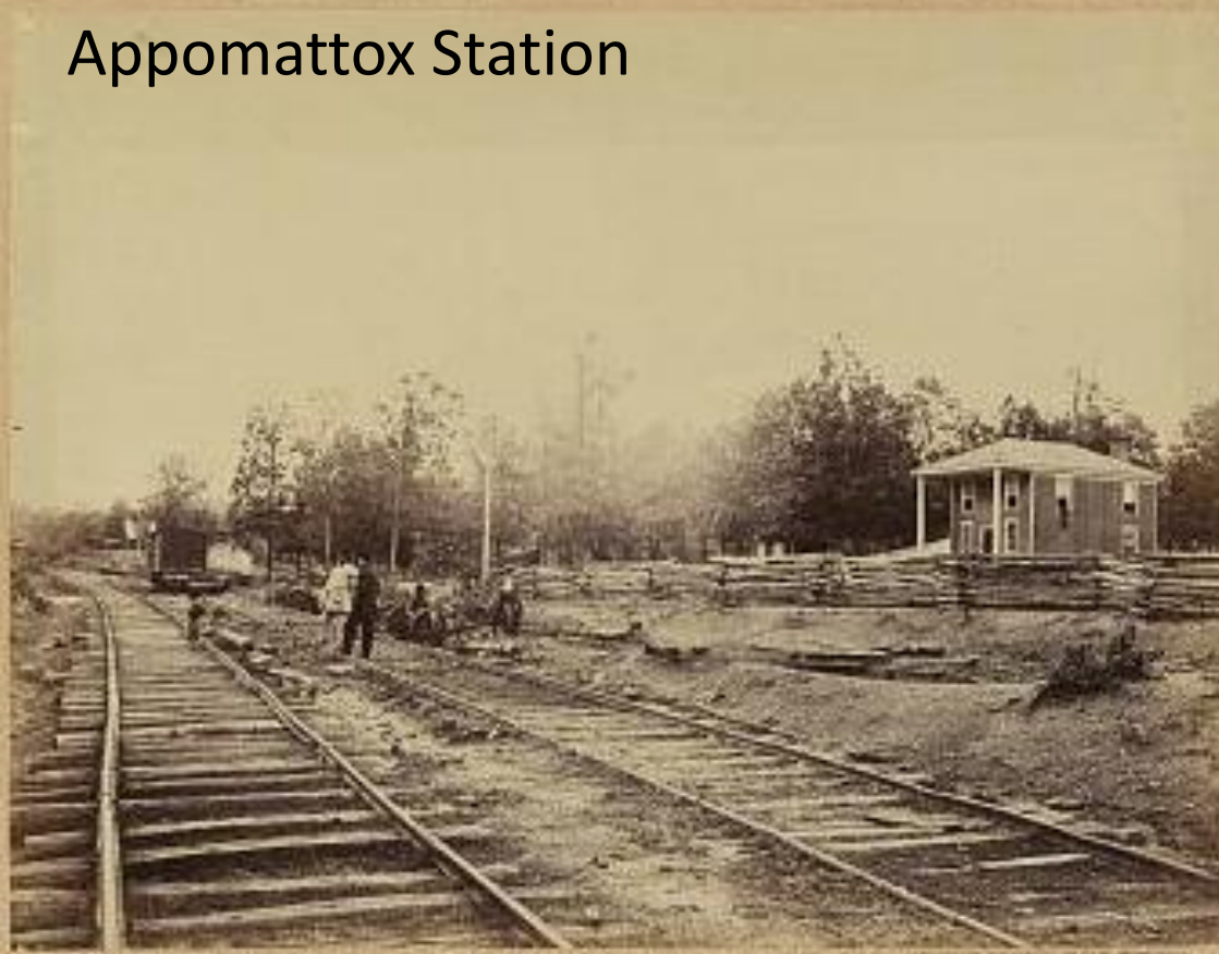
APPOMATTOX STATION, VIRGINIA.
